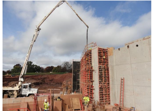
Figure 9: Concrete Pump Truck Courtesy of Gilbane Building Co.
