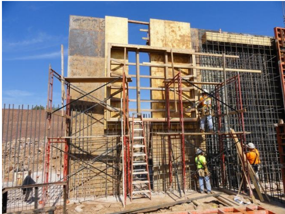
Figure 8: CIP Formwork Courtesy of Gilbane Building Co.
